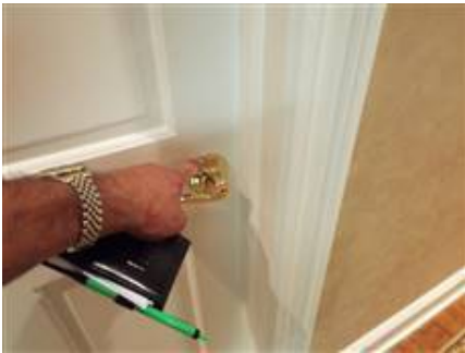
Photo 47-1 1st floor guest room.
