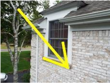
Photo 7-1 Area as viewed from the roof on the right side.
