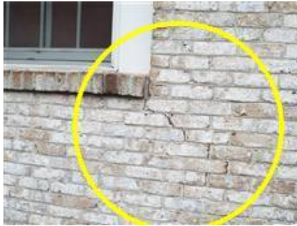
Photo 7-2 Close ups in next two photos.
