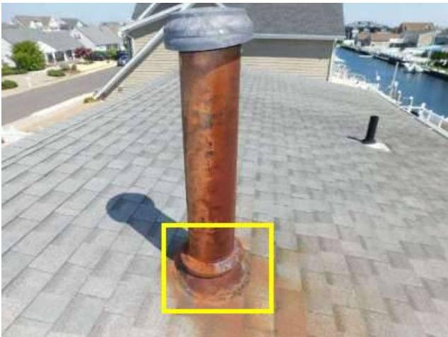
Photo 19-1 Close up of this area in the next photo.
