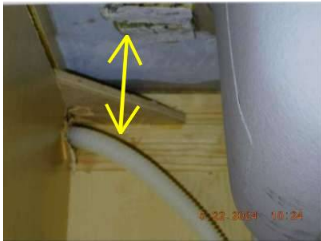
Photo 67-2 Ideally, the dishwasher drain line should be routed to the HIGHEST point underneath the countertop.
