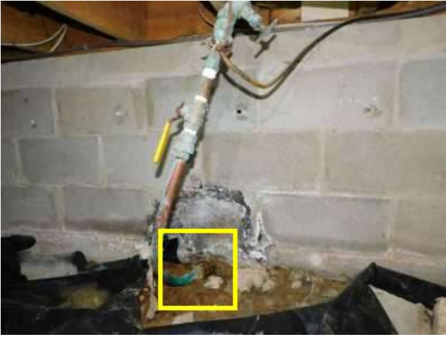
Photo 46-1 Close up of this area in the next photo.
