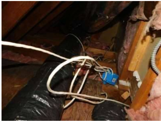
Photo 39-4 Knee wall attic space.
