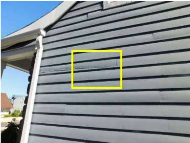
Photo 14-1 Close up of this area in the next photo.
