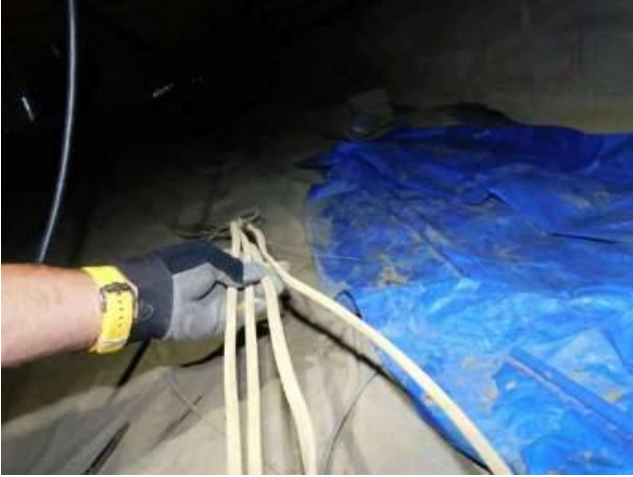
Photo 39-1 Crawl space here and the next 2 photos.
