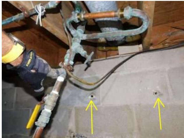
Photo 2-2 Drill marks seen in the foundation wall. Highlighted with the arrows.
