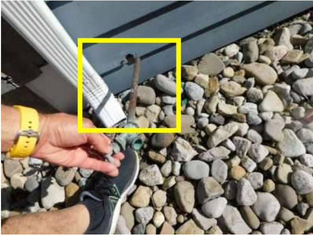
Photo 48-1 Close up of this area in the next photo.
