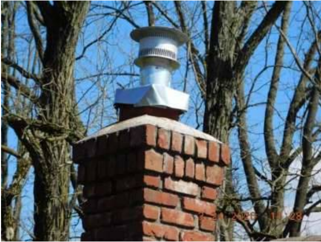
Photo 95-1 This is an example of a metal flue from a DIFFERENT property. No metal flue was seen for THIS property.
