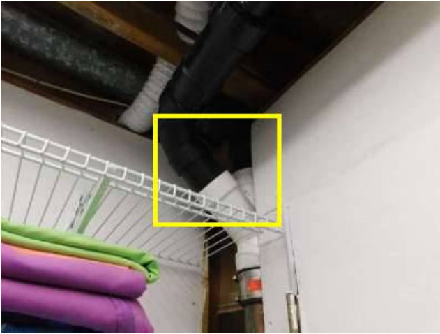
Photo 61-1 Close up of this area in the next photo. Laundry area.
