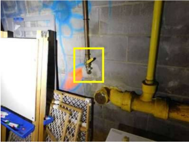
Photo 69-1 Close up of this area in the next photo.
