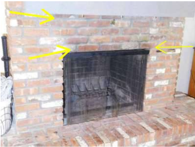
Photo 97-1 Note the darker shade of brick directly above the fireplace.
