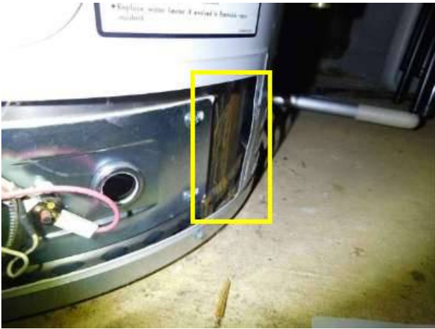
Photo 72-1 Close up of this area in the next photo.
