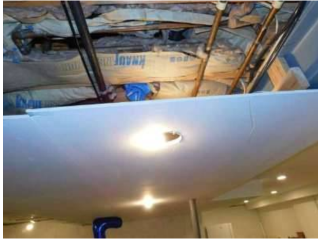
Photo 36-4 Close up of this area in the next photo.
