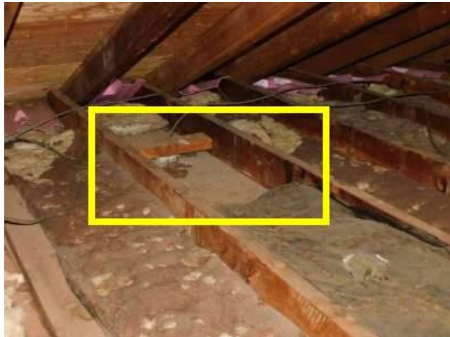
Photo 24-8 Close up of this area in the next photo.
