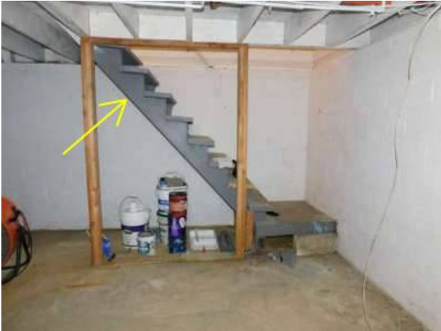
Photo 27-1 Close up of this area in the next photos.
