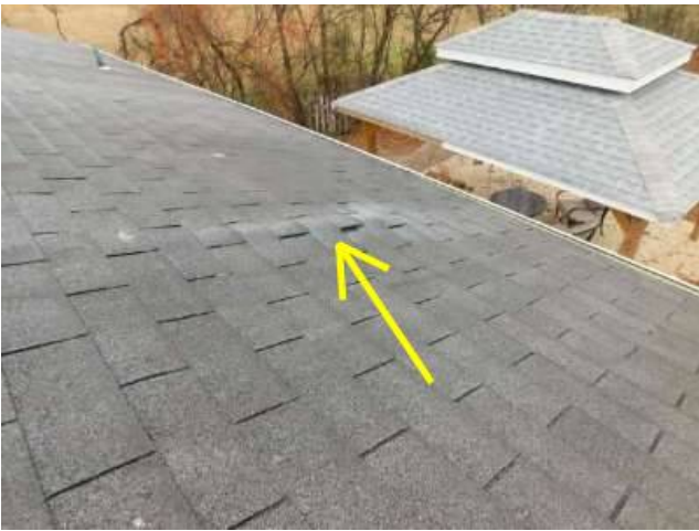
Photo 16-1 Close up of this area in the next photo.
