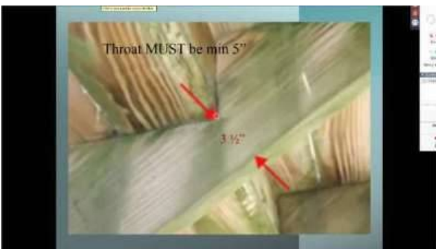
Photo 27-5 This slide is from recent training and shows that the stringer's shoulder must be, "min 5 inches."
