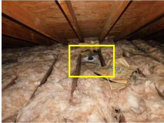
Photo 24-6 Close up of this area in the next photo.
