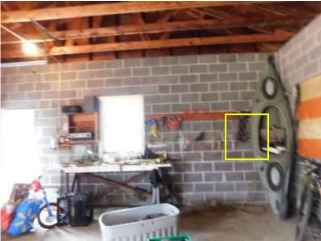
Photo 45-1 Close up of this area in the next photo.
