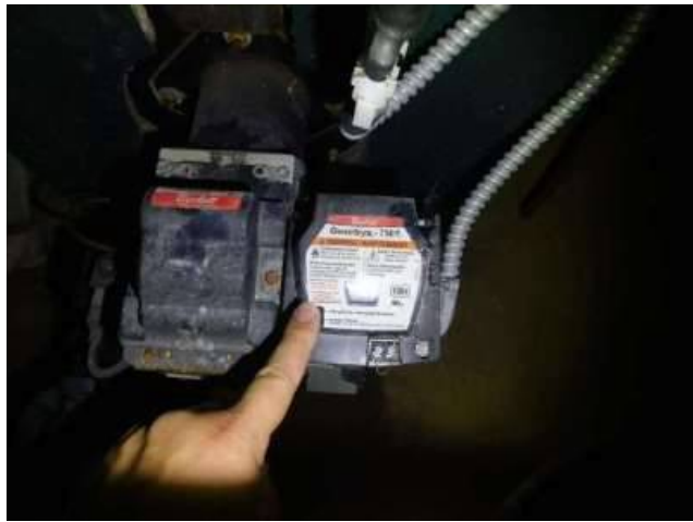
Photo 74-2 The light on this part of the boiler was blinking.
