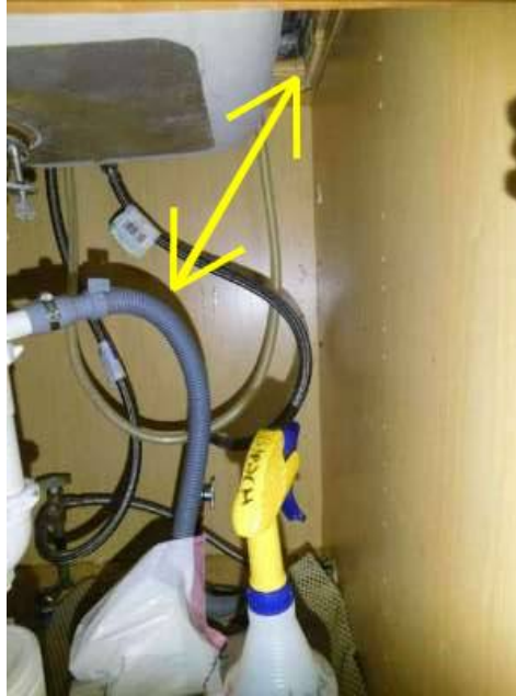
Photo 82-2 This is an example of a high loop from a DIFFERENT property. No high loop was seen for THIS property.
