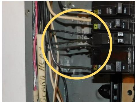
Notice the water as highlighted in both photos. Water is entering the panel as seen on the photo on the left and drops of water are hanging off the wires in the photo on the right.
