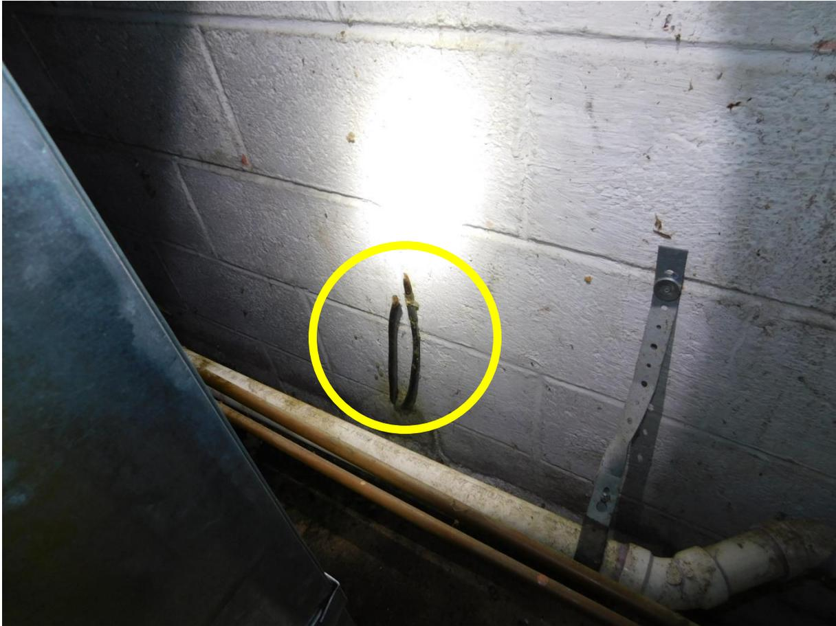
this photo, the copper tubes are now folded against the wall. Due to the fact that they are through the foundation wall the associated tank was most likely underground on the other side of the wall. I, as the inspector was not able to see under the ground so the client was urged to have an oil tank sweep done. From an inspection report perspective, this was identified as a, "Material Defect".
